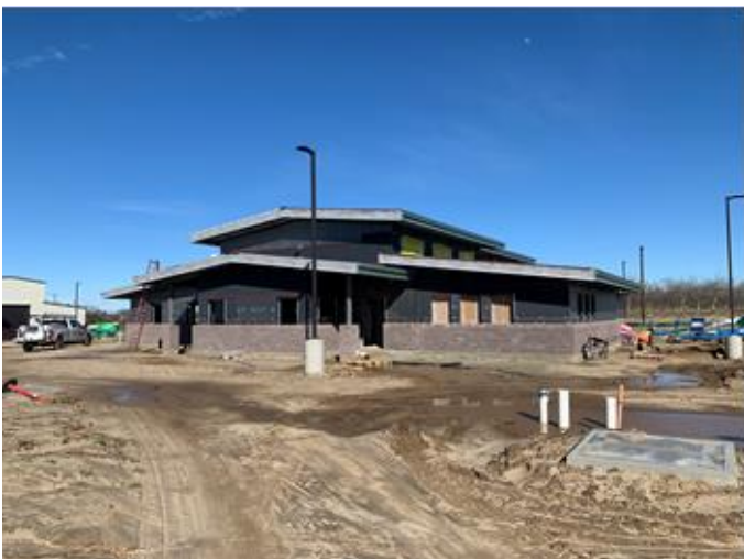
Administration and Operations Building
