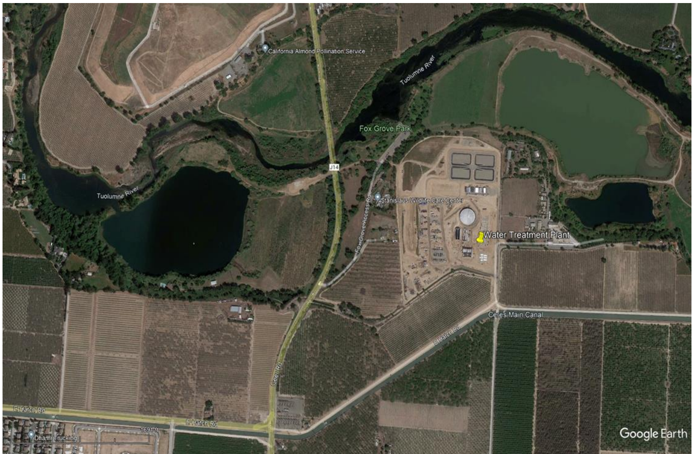
General Location of Water Treatment Plant
