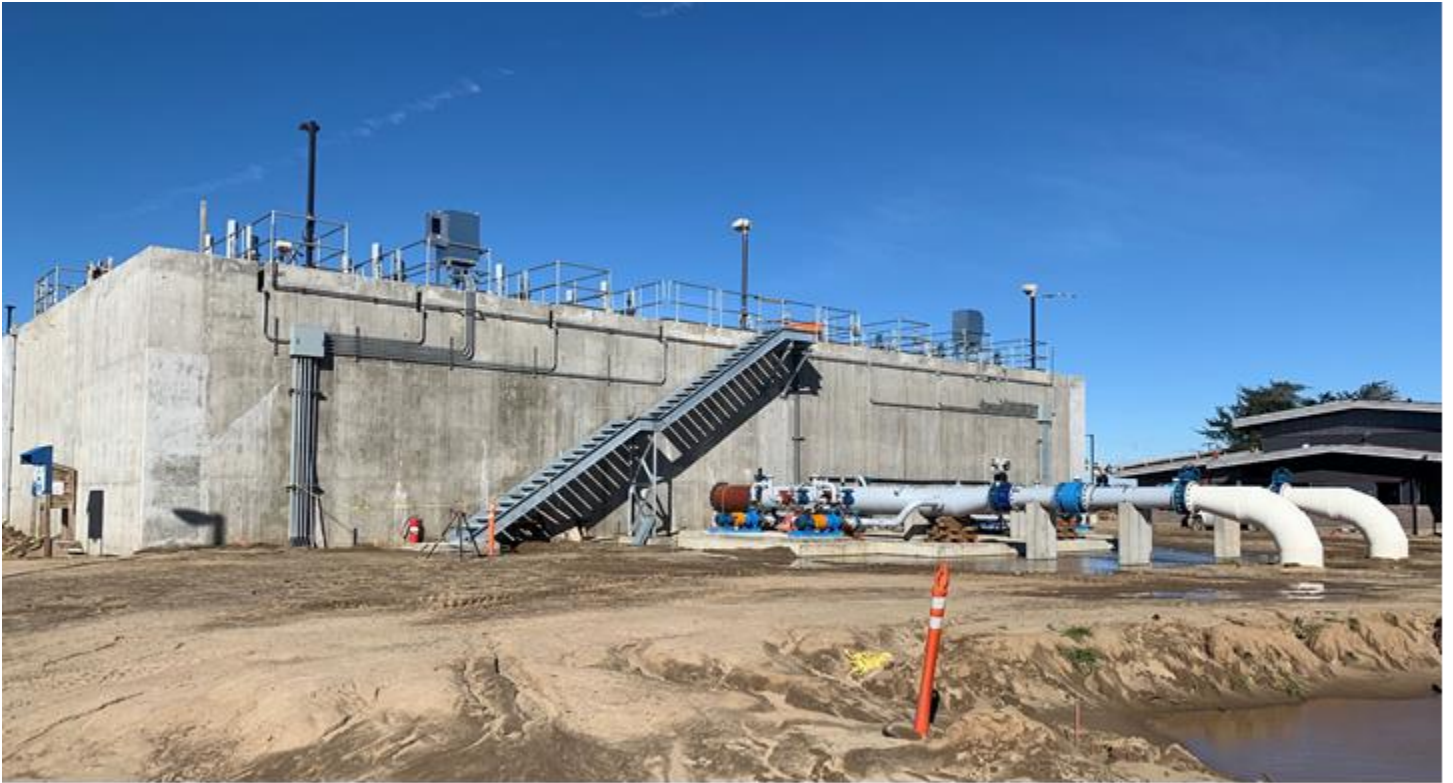
Flocculation and Sedimentation Basin
