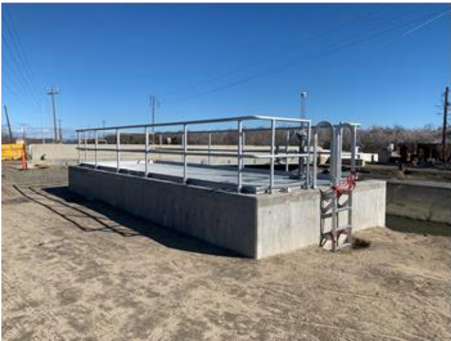
Ceres Main Canal Outfall Structure
