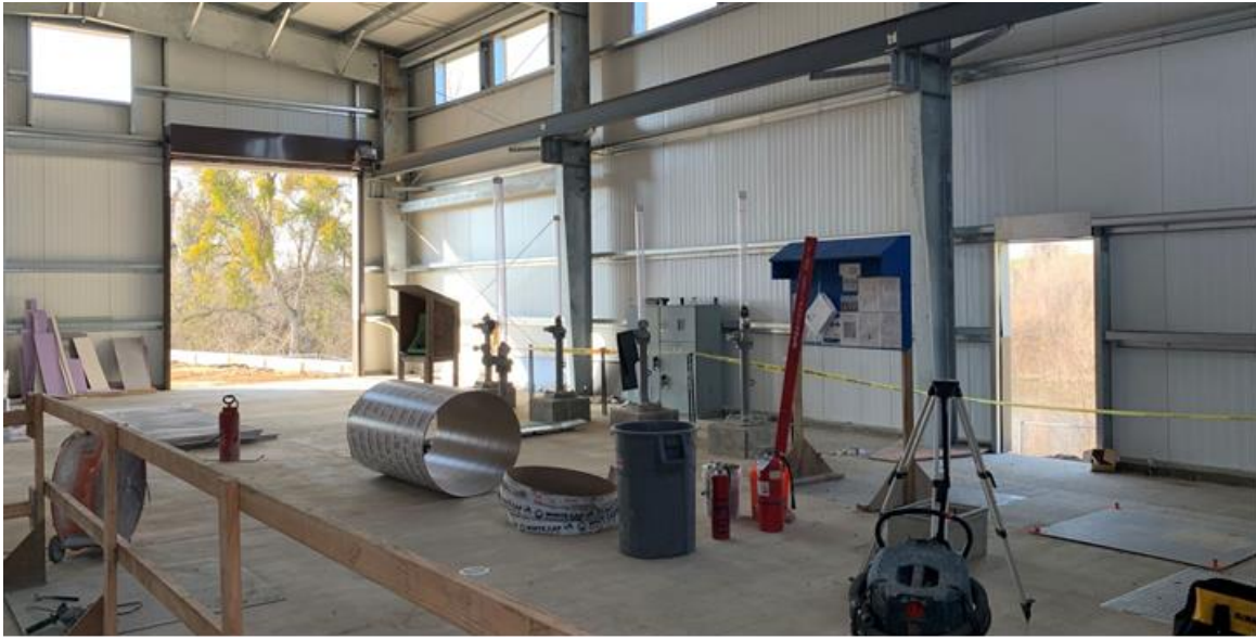
Interior of the Raw Water Pump Station Building
