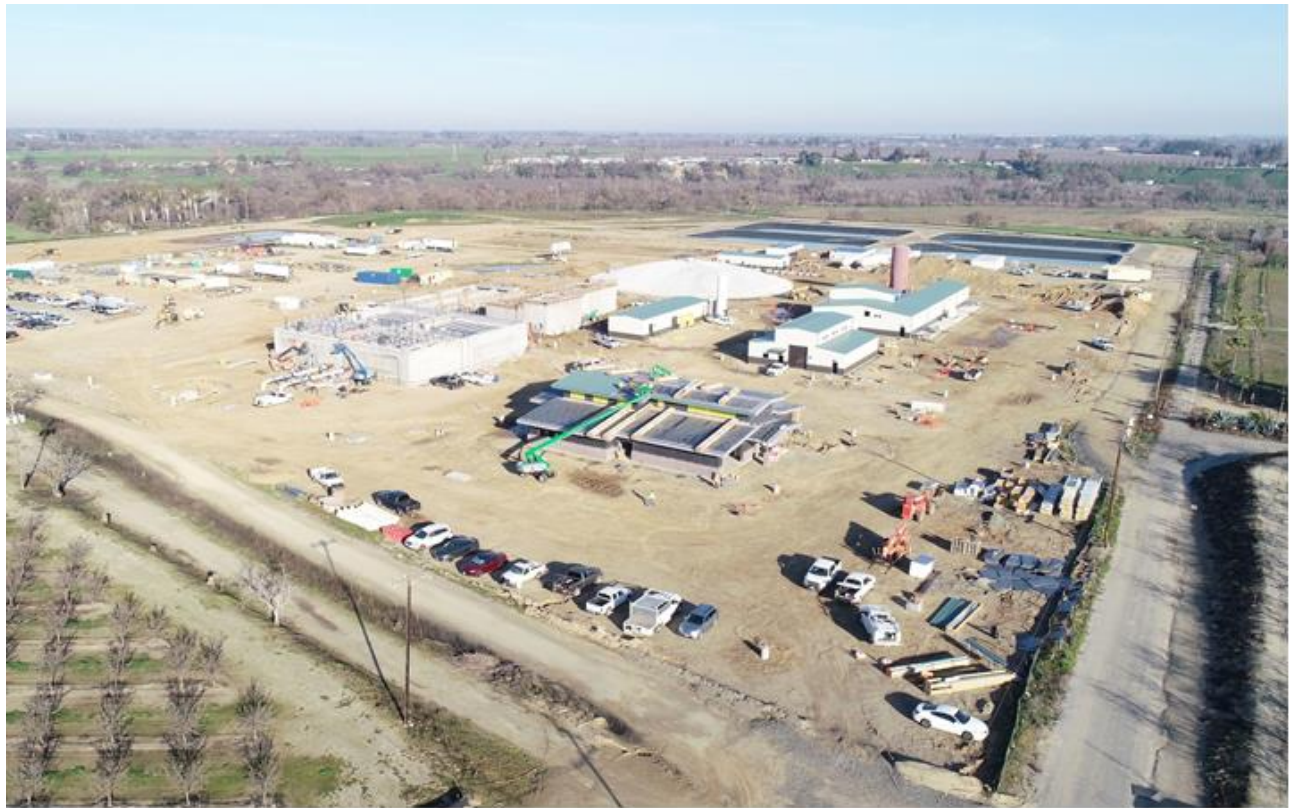
Aerial View of Water Treatment Plant Site (looking northwest)
